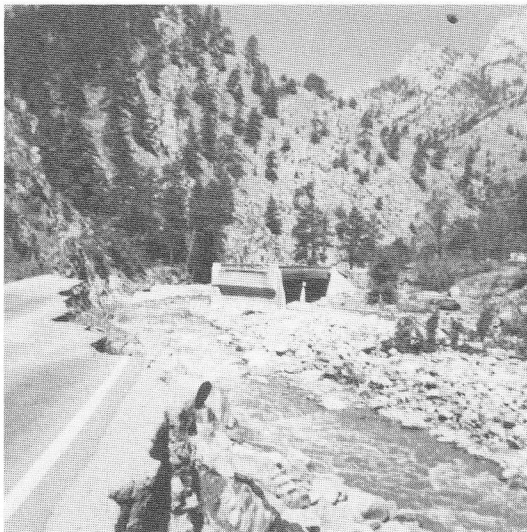
“In 1976, . . . the Big Flood scoured a wide, two-lane asphalt highway— this highway—completely out of the {Thompson} Canyon . . . here in the Narrows.” Photographs courtesy of the City of Loveland (CO).
